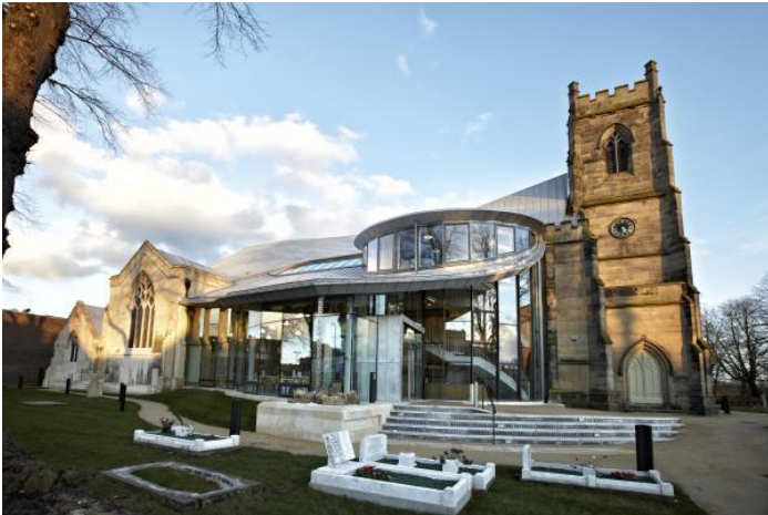
The rebuilt St Barnabas Parish Church, Erdington
