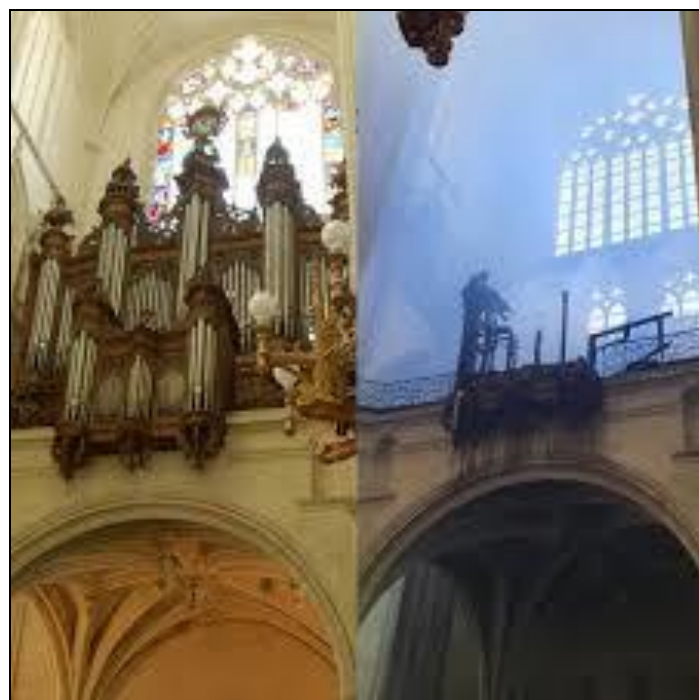
Nantes Cathedral organ – before, and after the devastating fire
