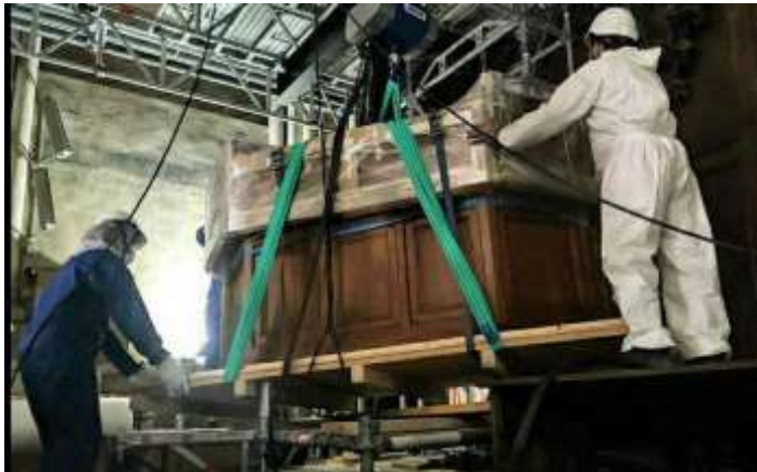
Notre Dame organ console being removed, August 2020
