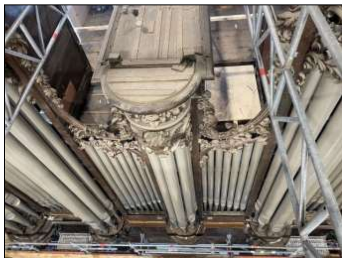
Notre Dame organ pipework – covering of lead monoxide dust
