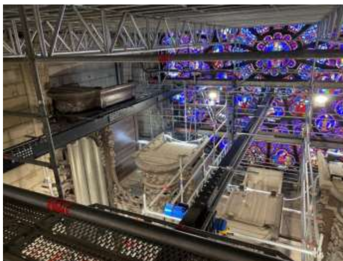
Notre Dame organ restoration – view towards West Facade Rose Window
